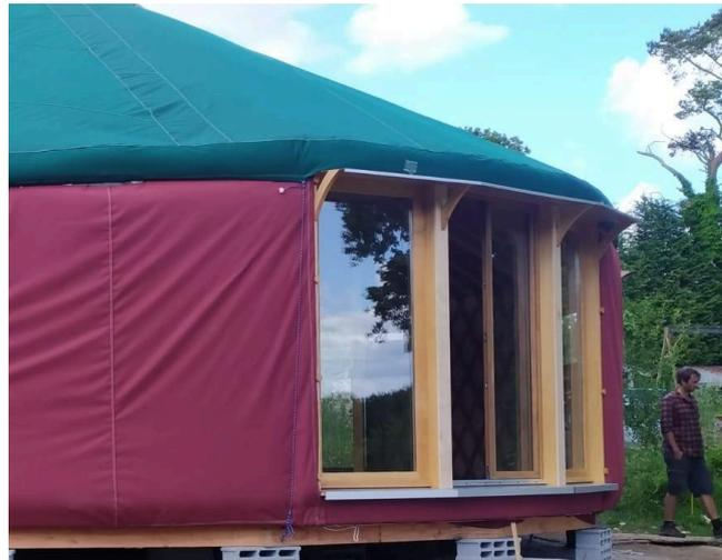
*PORTE DOUBLE ENTOURÉE DE DEUX CHÂSSIS VITRÉS FIXES – YOURTE DE Ø 10M*
