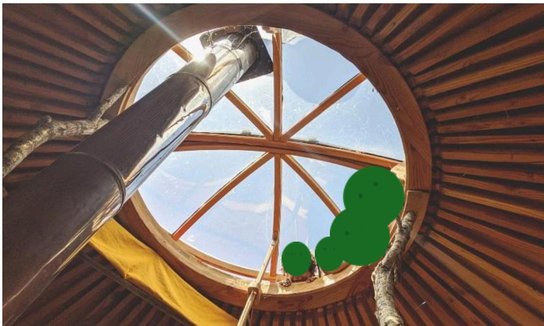
*OCULUS DOUBLE PEAU AVEC PASSAGE CONDUIT DE POËLE ET SYSTEME D'OUVERTURE*
